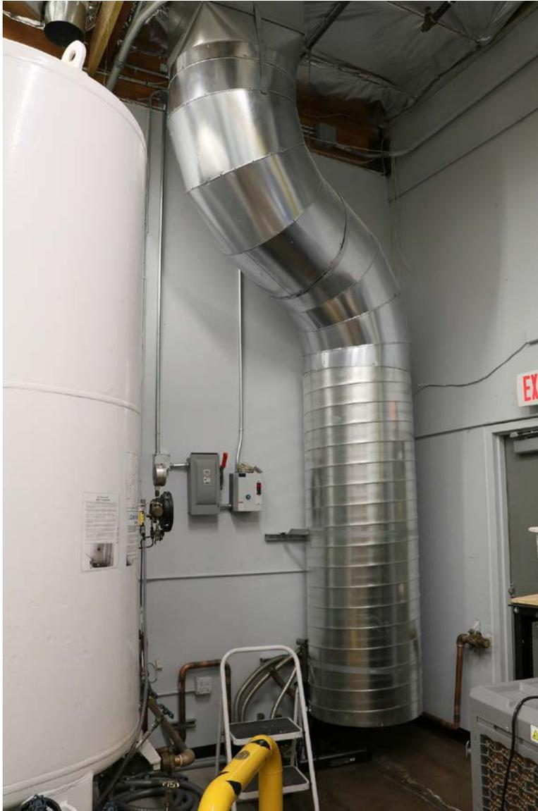
*Figure 20-32. One of several large ventilation ducts in Alcor's patient care bay. Fans on the roof are activated automatically if an oxygen sensor suggests a buildup of nitrogen in the air.*
